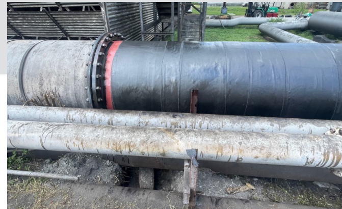
Figure 3 The composite repair reinforced the water line
