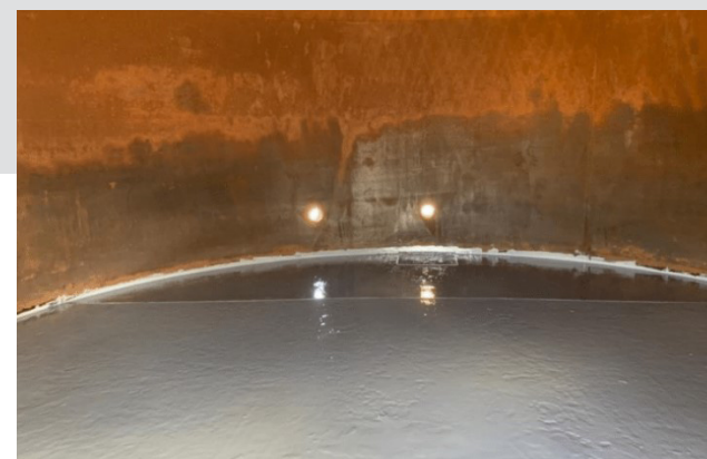
Figure 3 Chemically resistant epoxy novolac coating system
