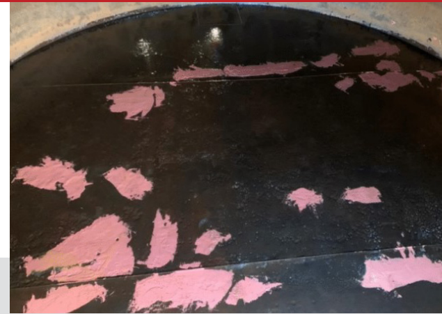
Figure 1 Repair putty filled in pitting
