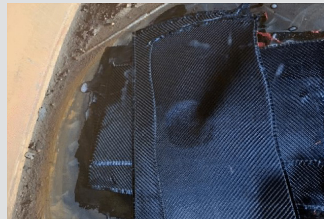
Figure 2 Carbon fiber patches addressed through-wall failures
